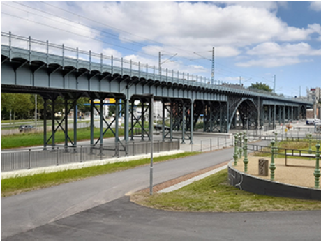
Image 1 Chemnitz steel viaduct
