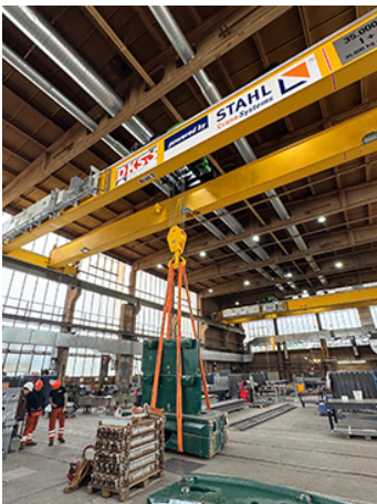
Image 3 Acceptance inspection by STAHL CraneSystems
