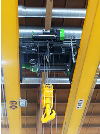
Image 4 Hoist in Crane
