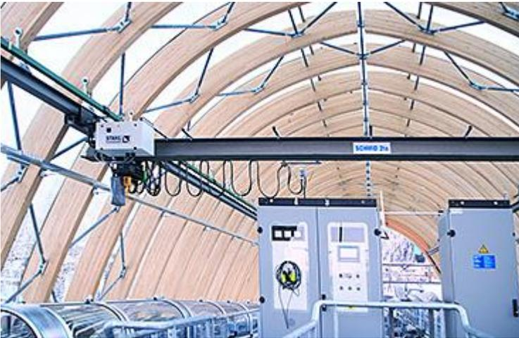
Detailed view with ST 20 chain hoist of STAHL CraneSystems. A colour was chosen for the crane girders and crane track that came closest to the hot-dip galvanised crane track suspensions.
