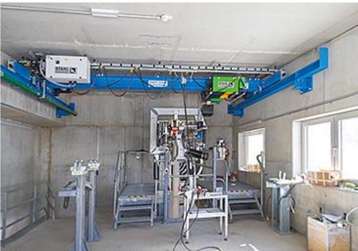
Even in the maintenance section of the middle station, every millimetre counts. With the very restricted height, the STK 50 chain hoist with extra-short headroom trolley makes very small starting dimensions possible.
