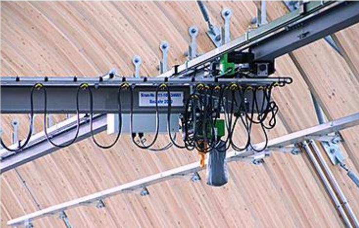
For the suspension of the crane track, a solution was developed involving a larger cross section in the attachment area on the laminated wooden beams and the crane track, while it tapers out in the middle.
