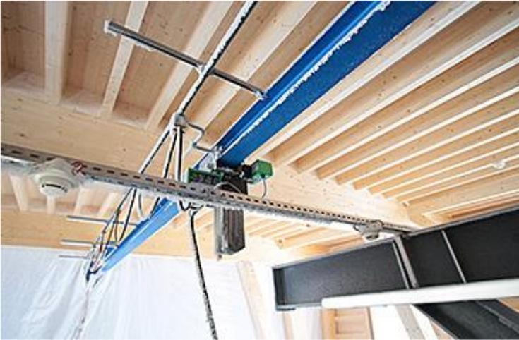
The roof of the mountain station is supported by laminated wooden beams. The monorail suspension crane with a load capacity of 1.6 tons must be mounted in horizontal suspension when the roof is sloping.
