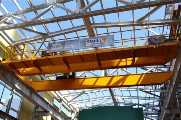
The cranes and hoists were assembled before completion of the hall roofs to facilitate the work.
