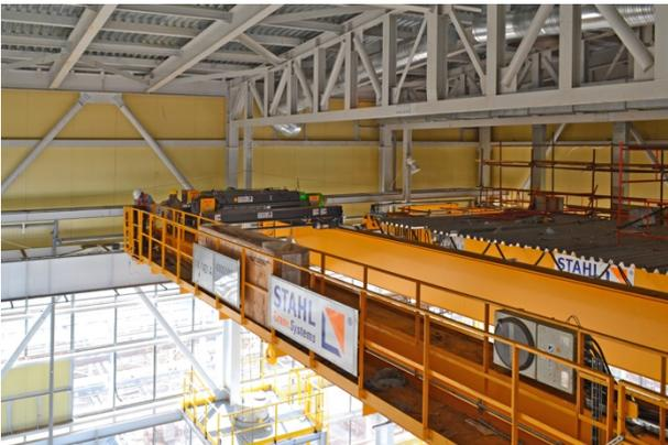
To ensure smooth operation of the plant, there are a total of 11 cranes, 6 electric wire rope hoists and 30 manual chain hoists from STAHL CraneSystems in use.
