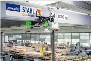
Enclosed conductor lines provide a safe and elegant power supply along the crane bridge.
