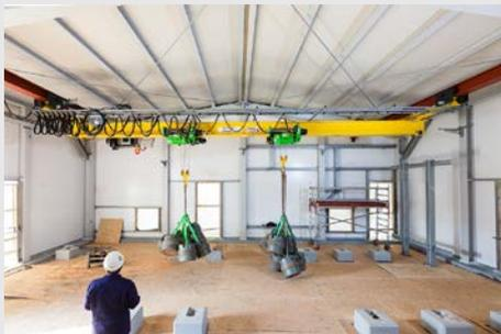
There's no explosive gas here yet: the customised crane on the construction site of the metering and control station is tested with 125 % of the permissible rated load of 6.4 t.
