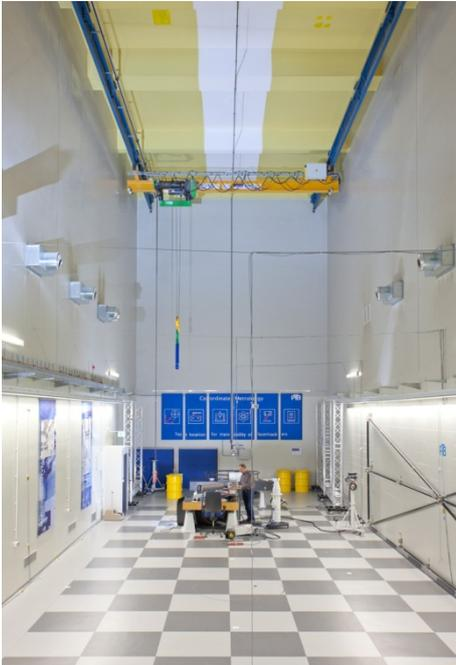
The unusual shape of the room is owed to its previous use as a reactor. Nowadays laser trackers are tested and calibrated here. A suspension crane from SMI tech travels on the old crane runways.
