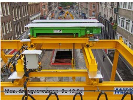
Roofs protect the hoists from rain and dirt.
