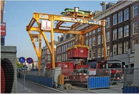
The frequency-controlled ASF7 wire rope hoists load the containers onto lorries quickly and precisely.
