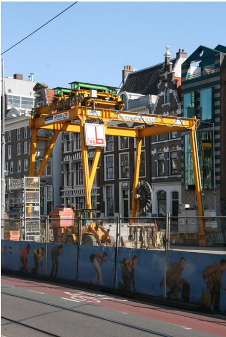
A portal width of 8 metres enables safe loading and unloading operations in spite of concurrent car traffic and the continuing operation of the existing tram line.
