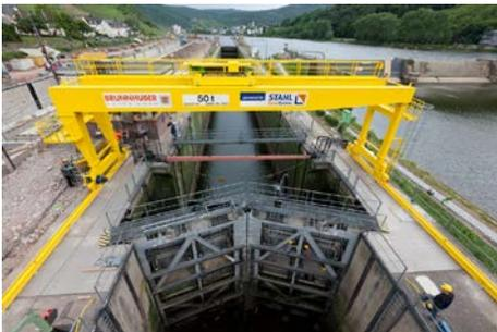
The fully erected portal crane at the aft lock gate. Maintenance work is carried out on the lock gate while the crane is being erected.
