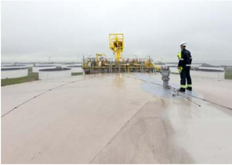
A maintenance crane is positioned on each tank to lift the liquefied gas pump out of the tank and set it down outside, adjoining the tank.
