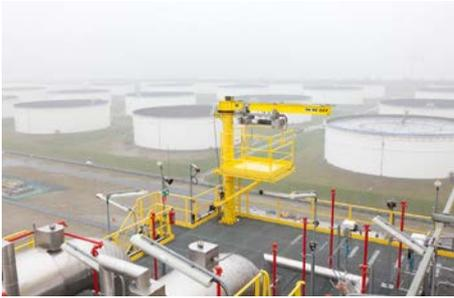
These auxiliary cranes with wire rope hoists type SH 30 ex are approved for explosion protection zone 2. A hoist brake with manual release permits the load to be lowered safely even in a power cut.
