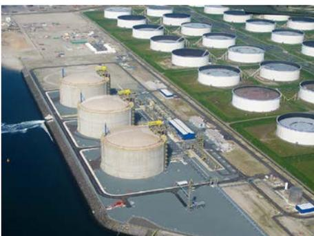
The GATE terminal in the Port of Rotterdam comprises three LNG tanks with a total volume of 540,000 m<sup>3</sup> liquefied gas.
